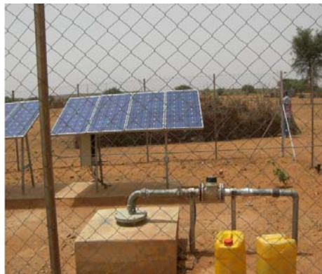
Left-AMG clusters five meters below the dam=hydraulic pressure Center-solar pumping Right-free flowing water from an artesian borehole All are sources of alternative energy to be used by the AMG
